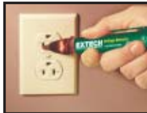
Line outlet testing
