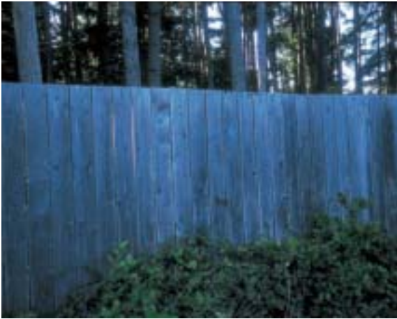
Exposure to weather causes graying.
