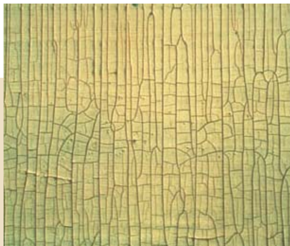
Alligatoring (courtesy Behr/Rohm & Haas).
