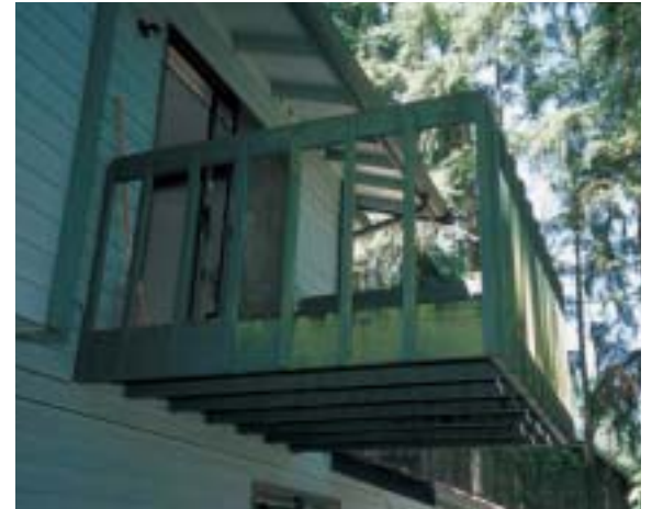
On this deck, mildew grows only outside the drip line of the roof.
