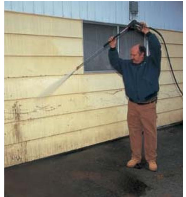
Set the pressure washer on a wide fan and aim downward if you are working on lapped siding.
