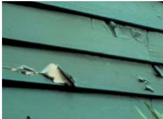
Peeling (courtesy Behr/Rohm and Haas).
