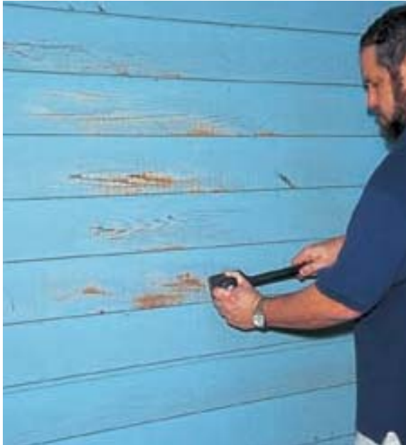
Use scrapers or a wire brush to dislodge loose paint.
